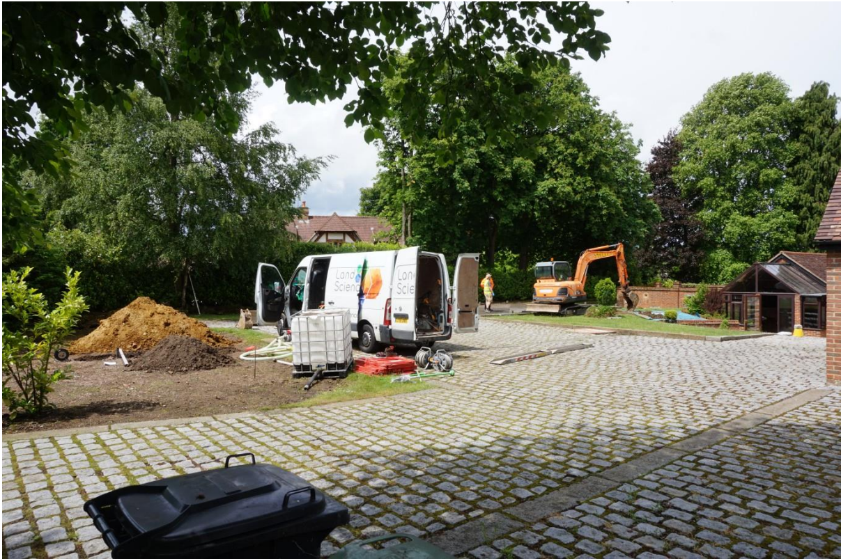
Plate 1: Looking west-north-west at the site. Trench 3 is visible on the left, Trench 2 is located by machine and Trench 1 is located behind the wall obscured by machine bucket. Note house entrance on the right is located on lower ground
